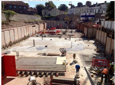
The picture above gives a view of the basement section of the new building with two out of three sections of the basement floor slab cast in place
