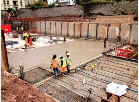
The picture above shows how the basement floor slab is cast in sections on top of a layer of re-enforcing mesh, using ready-mix concrete pumped down from road level.
