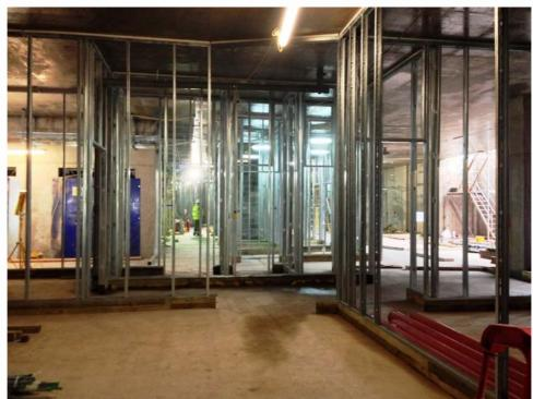
This picture gives a glimpse into the basement of the new hospital and shows the metal framework for the partition walls being erected.
