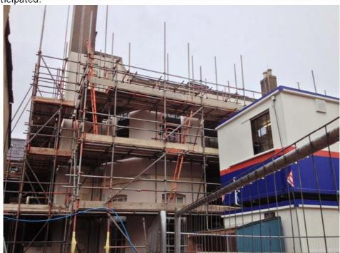
The picture above shows the scaffolding going into place on the rear elevation of the Grade II\* listed building to enable the external refurbishment to commence
