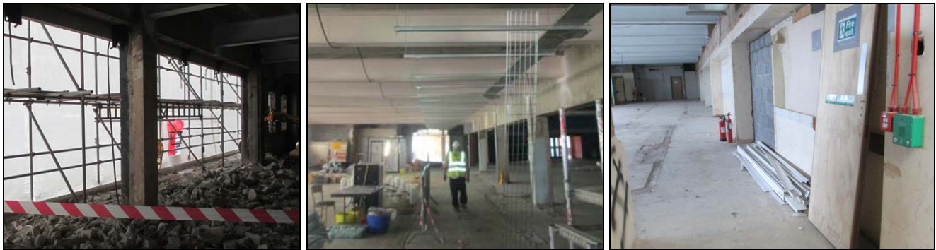
Phase 2 refurbishment work has now started!
