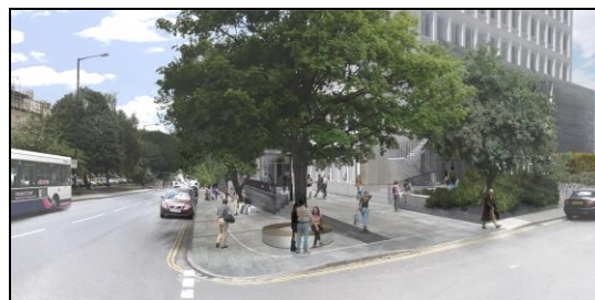
Concept view of the refurbished building and new entrance to Queen's Road (Feilden Clegg Bradley Studios)
